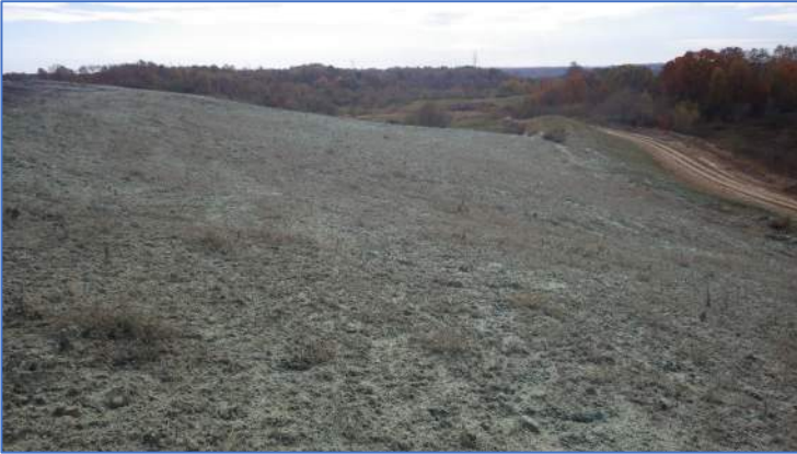
Photo 4 Southwestern slope of Phase 1, looking south.
