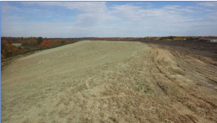
Photo 6 View of western crest of Phase 1, looking north.
