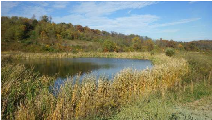
Photo 35, Point 30 The Interim Leachate Collection Pond as viewed from the southwest corner.
