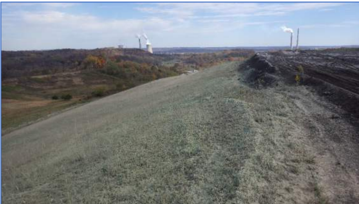
Photo 11 Top of CCRs on northern edge of Phase 1. Slope is hydroseeded.
