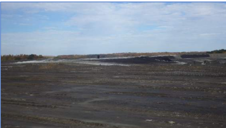
Photo 12 Chimney drain in northern Phase 1.
