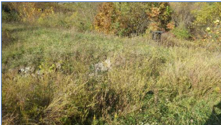
Photo 36 Overflow structure near Interim Leachate Collection Pond.
