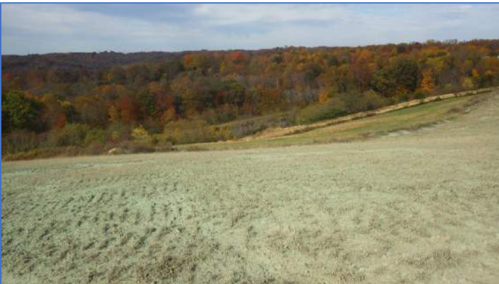
Photo 15 Outer slope of the western edge of Phase 1 and the northern access road in background.
