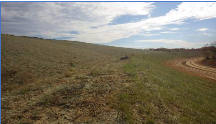
Photo 2, Point 1 Southwest outer slope of Phase 1. Limit of bench with new hydroseeding.
