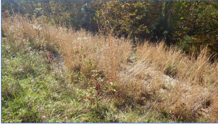
Photo 28, Point 28 Possible scarp on northwest side, exterior slope of the West Sedimentation Pond.
