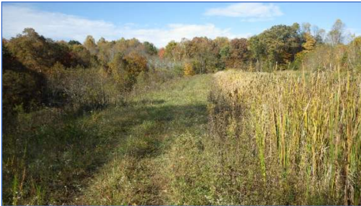
Photo 26 West dike crest of West Sedimentation Pond. Area is heavily vegetated.
