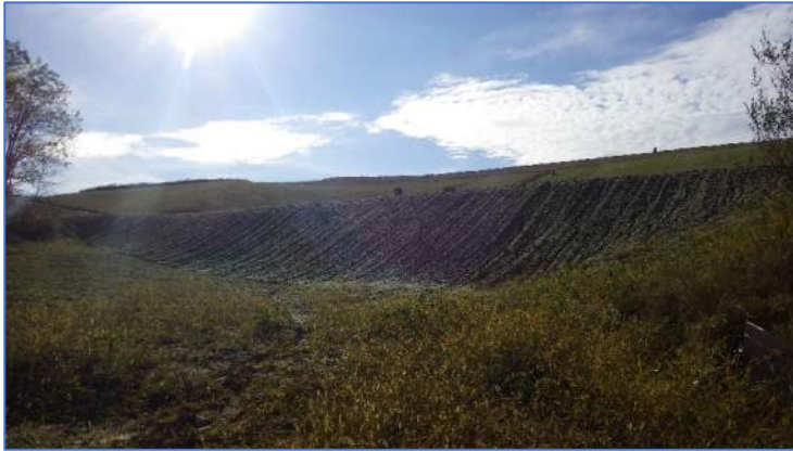
Photo 34, Point 30 Eastern toe of Phase 1 near the Interim Leachate Collection Pond.
